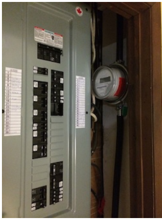
The kWh counter provided by roulezelectrique.com and the new panel 200A
